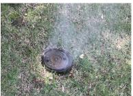
The smoke should not enter your home or business if it is properly plumbed, vented, and the water traps contain water. If smoke does enter a home or building, it will clear within 30 minutes with proper ventilation.
